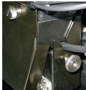
Figure 7-74: UV-lamp cable after replacing the assembly
