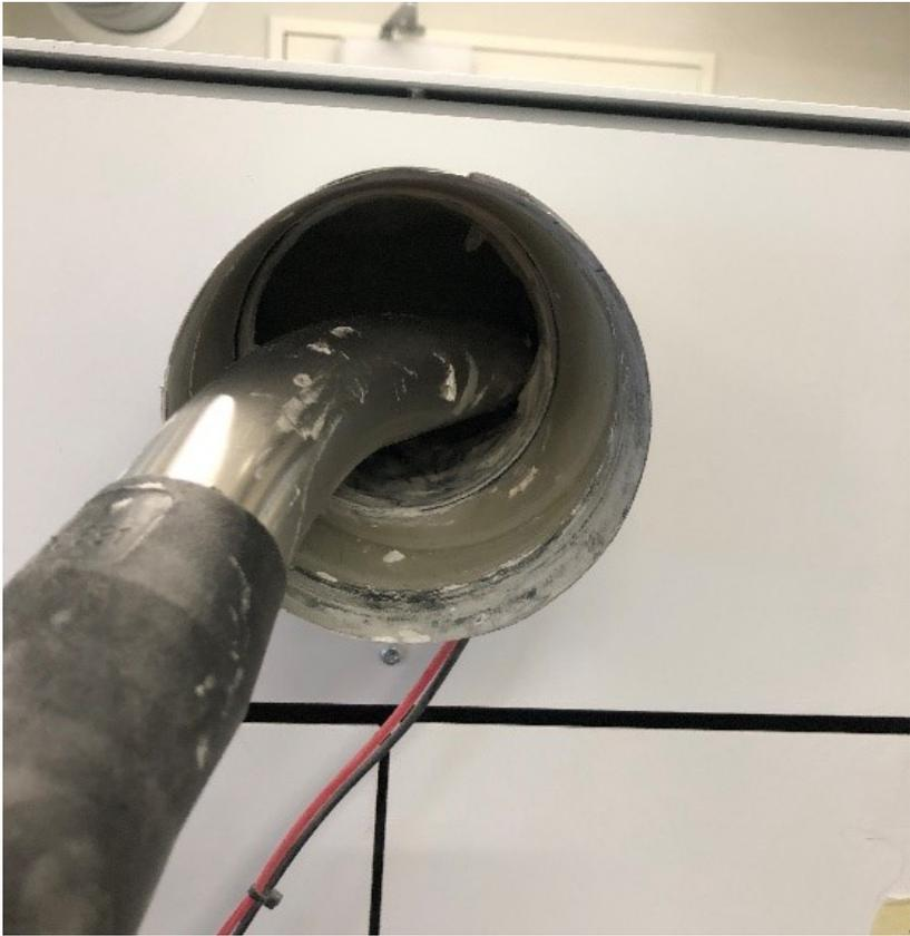
3. After cleaning, the extraction outlet (left) and the tube connection from waste cyclone separator (right) should look as shown in Figure 80.
