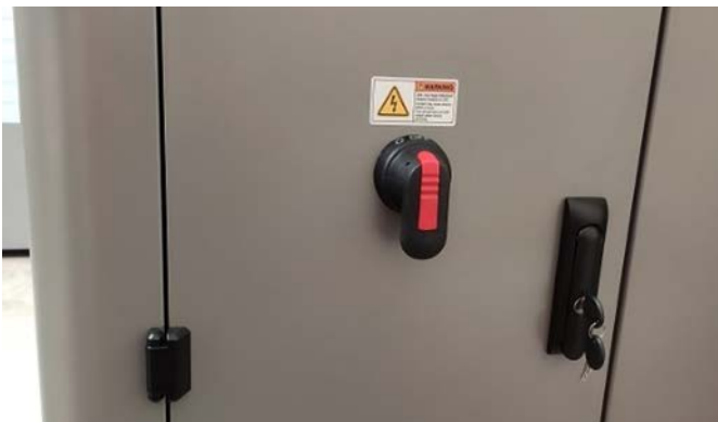
Figure 1: Power Isolator in the ON position
