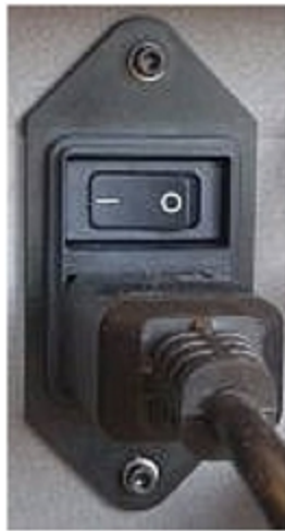
Figure 6-2 Main power switch and cable
